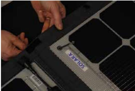
Stick the wire rope through the hole in the module.
