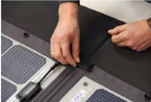
Fix the module with the velcro in the middle. This reduces the risk that wind gust lifts up the panel.
